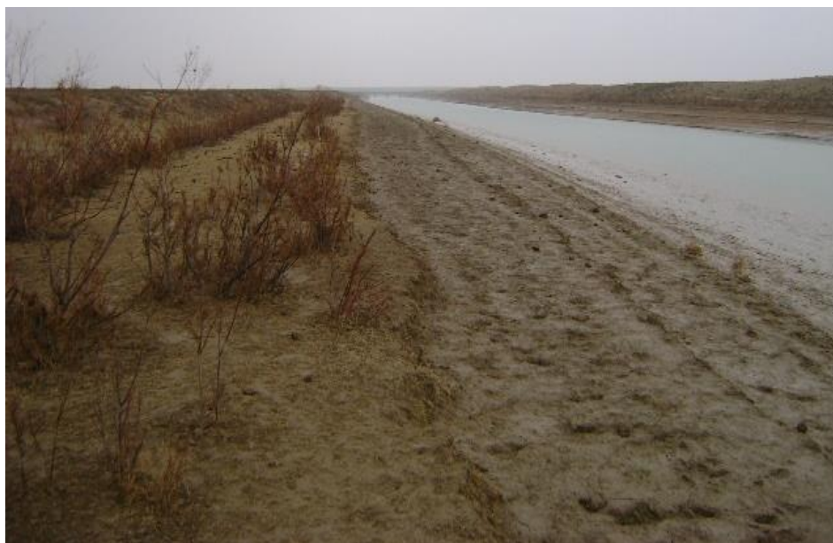
Figure 1. General view of Mirishkor canal at PK 180 station
