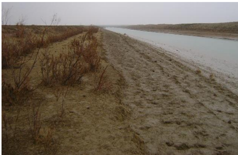
Figure 1. General view of Mirishkor canal at PK 180 station
